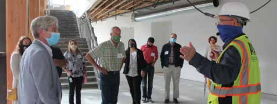
Prospective donors and community leaders participate in a tour of the King City Education Center expansion under construction on Nov. 18, 2020.
