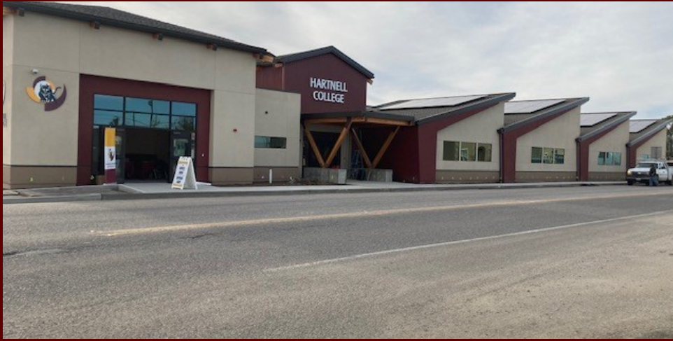
CASTROVILLE—Merritt Street Entrance
