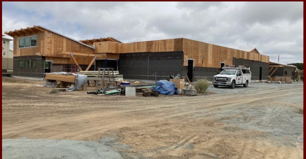
CASTROVILLE Education Center—Work commenced to the application of stucco paper for the exterior finish application June 30, 2021
