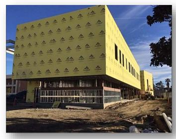
In Castroville, installation of underground utilities is wrapping up, slabs have been poured in some sections of the building and framing will start soon.
