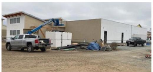
In Castroville, the stucco finish coat has been applied to the exterior (pictured left) and skilled trade workers are installing electrical, mechanical, plumbing systems as well interior finishes. Curb, gutter and paving work are close to completion as well. The center is scheduled for completion by early 2022.
